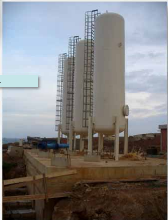
Hydropneumatic tanks
