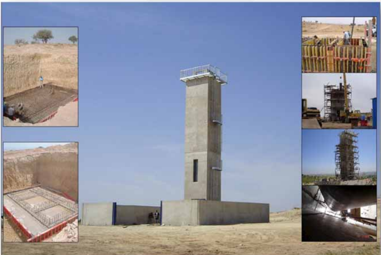
Hydraulic Disconnection Tower, against Water Hammering
